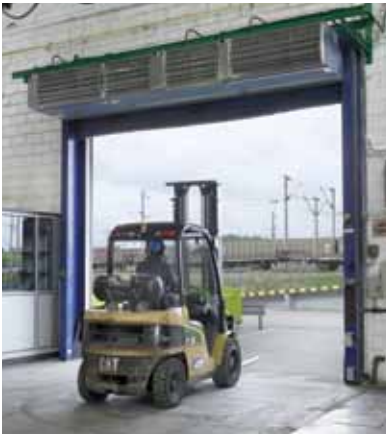
During loading and unloading the door remains open, without the indoor climate being disturbed.
